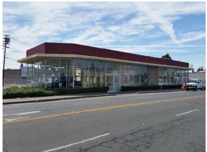
View from Georgia Street of the entire facility.
