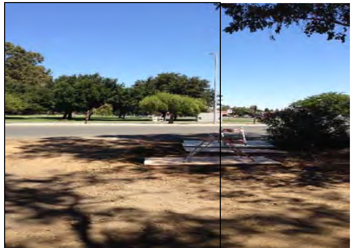
Pad for switch gear has been cleared.
