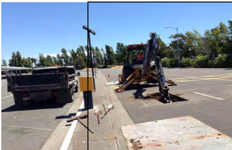
Pull box being excavated.
